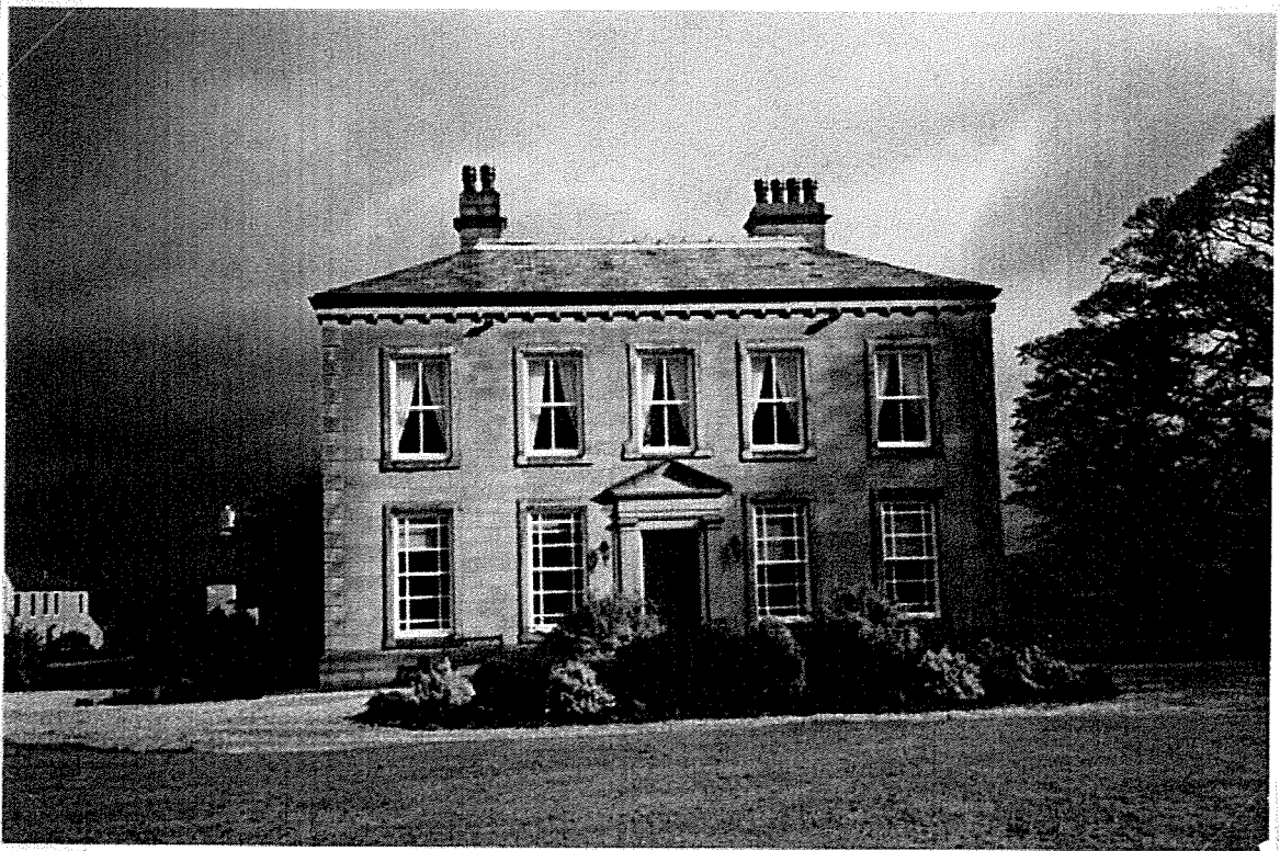
a. Front (Northward) View of New Clayton Hall
