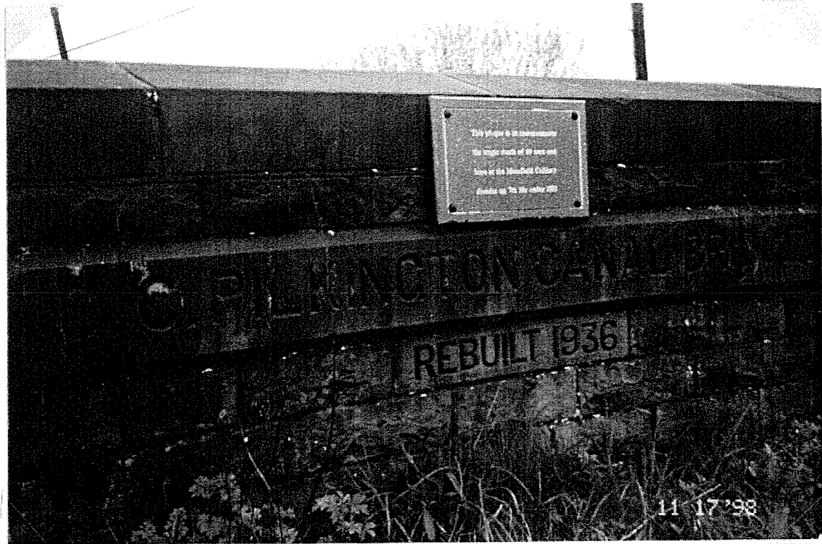
b. Bridge Across Leeds and Liverpool Canal for Highway A678, Near Site of Moorfield Pit Disaster (Note plaque, described below)
