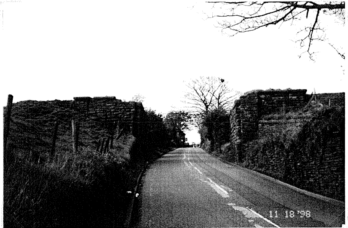
b. Bridge Abutments on Roman Road for Former Hoddlesden Railway Branch
